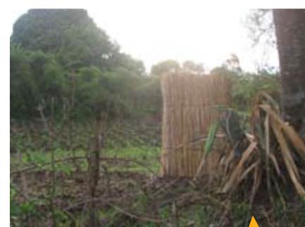
An open pit latrine sheltered with reeds. With time the reeds which are exposed to the elements of sun and rain rot. This structure therefore has to be reconstructed every so often to provide privacy.
